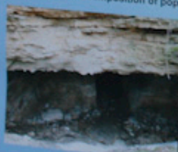
Entrance in Hagieni' Tunnel
